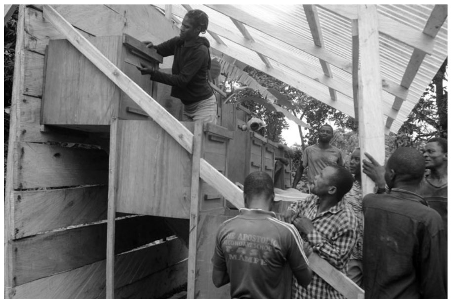
Installation of fermentation boxes for cocoa
