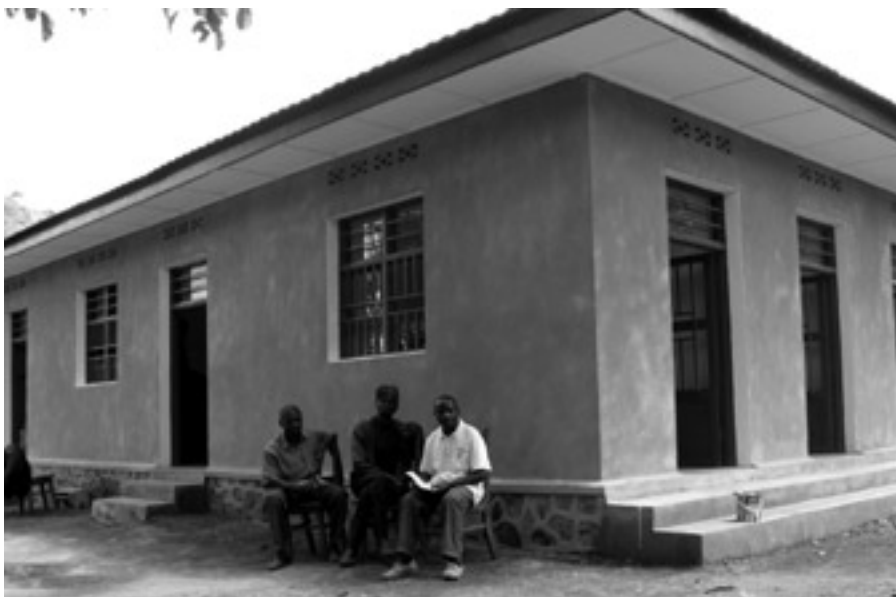
The newly constructed patrol post
